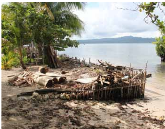
Building protective sea walls using coral reef that has been blasted is now a common practice in some of the islands off northern Papua New Guinea. Investing in the integrity of the coral reefs and surrounding mangroves is likely a much more cost-effective defence against the coming impacts of climate change. (Photo by James Watson)
